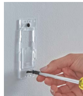
Install wall plate bracket
